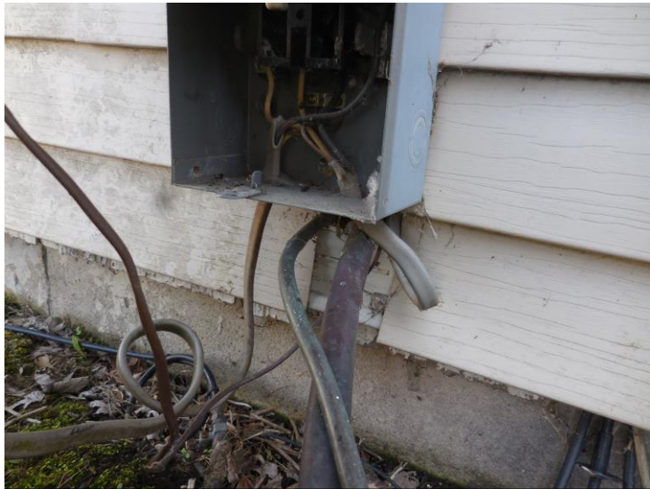
Non-professional wiring was found at the circuit for the central AC system.
